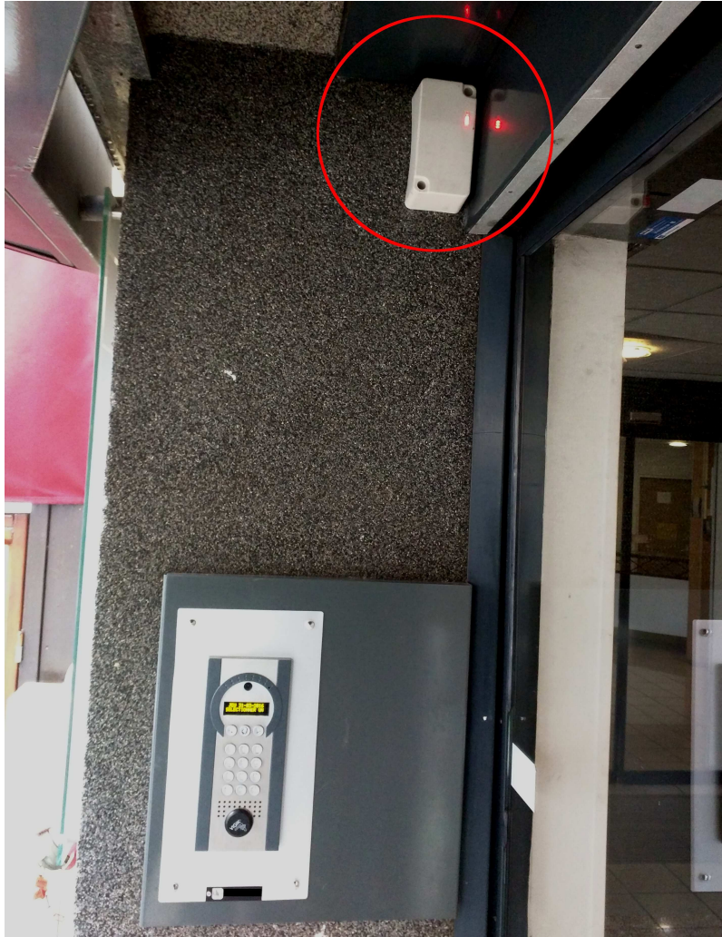
Figure 2: 3G block of an Intratone intercom
